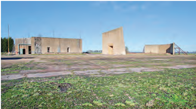
Wide view of K2 and its two blast walls
